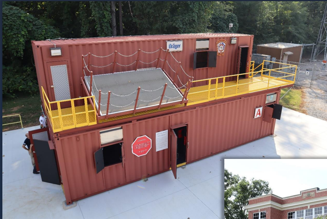
Completion of Live Burn Structure at Henley Fire Training Center
