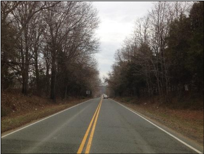
Photograph 11: Existing Ashland Road Two-Lane Cross Section
