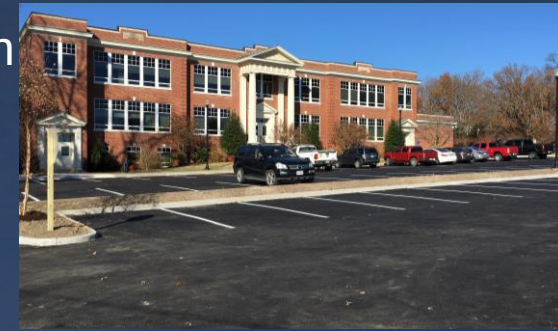
Administration Building Parking Phase I Expansion Completed
