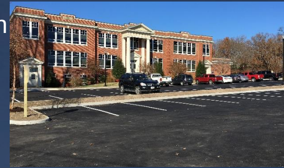
Administration Building Parking Phase I Expansion Completed
